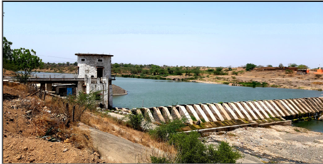
Fig.1: Intake Well at River Kunda near Santoshi Mata Mandir, Khargone
