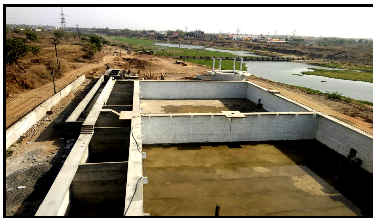
Fig. 8 & 9: STP of 17.6 MLD Capacity under construction at Khargone
